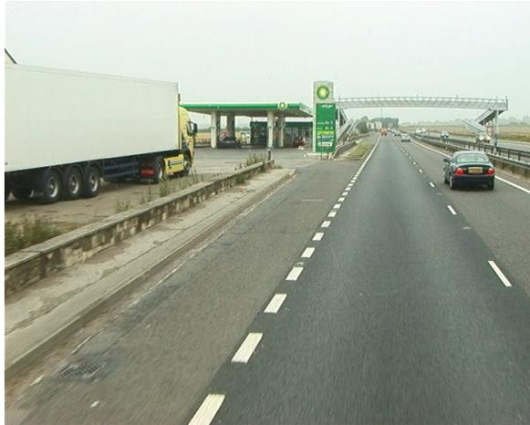
**Figure 1 Example of poor junction design for a busy access on to a 70mph road**
